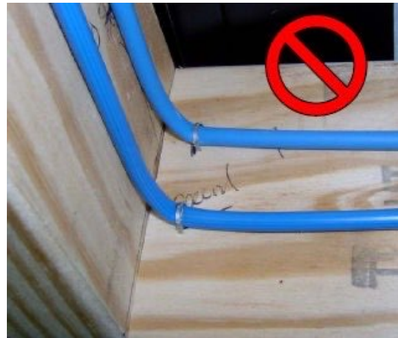
Figure 6 - Incorrect Procedure for Stapling Drop Cable in Corners
