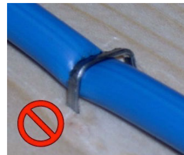
Figure 4 - Drop Cable with Flat Crown Staple
